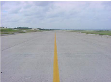
**TAXIWAY CENTERLINE MARKING:** Solid yellow line used to designate the center of the taxiway.
