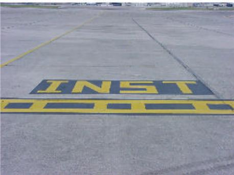
**INSTRUMENT HOLD LINE:** These lines consist of two parallel solid yellow lines with vertical stripes and the letters "INST" stenciled on the movement surface facing the driver. Instrument hold lines are located on taxiways Alpha, Bravo, Echo, and Foxtrot.
