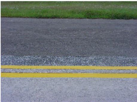
**EDGE OF STRESSED PAVEMENT MARKING:** A double yellow line used to mark the edge of the pavement stressed to support aircraft.
