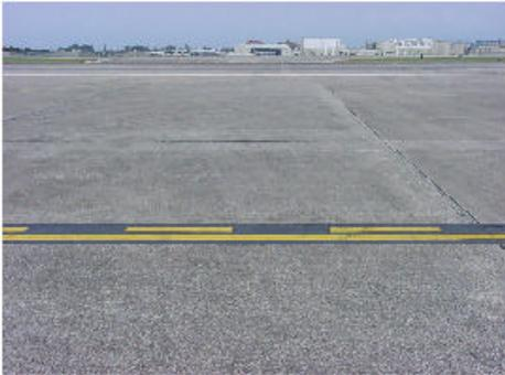
**Hold line:** A solid yellow line adjacent to a dashed yellow line, located 100 feet from the edge of the runways, helipads, and the VTOL pad. Vehicles and aircraft must contact the control tower and obtain permission prior to proceeding beyond the hold line.
